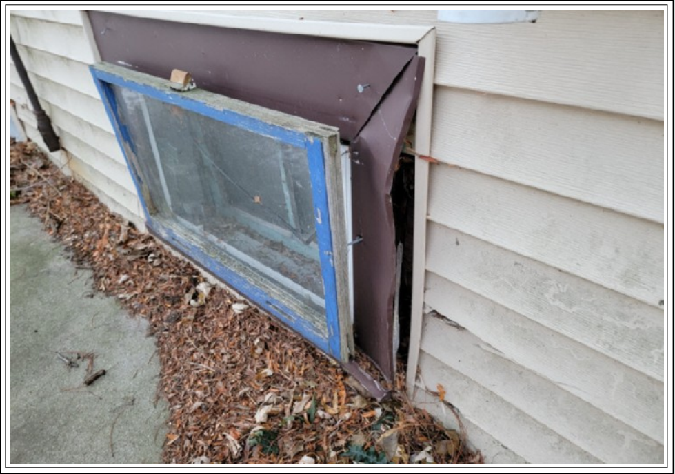
Basement Window Possible vermin/exterior elements infiltration
