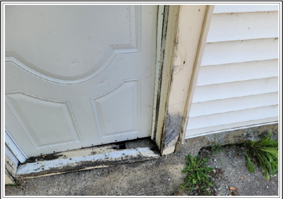
Defective Door Sills/Jambs
