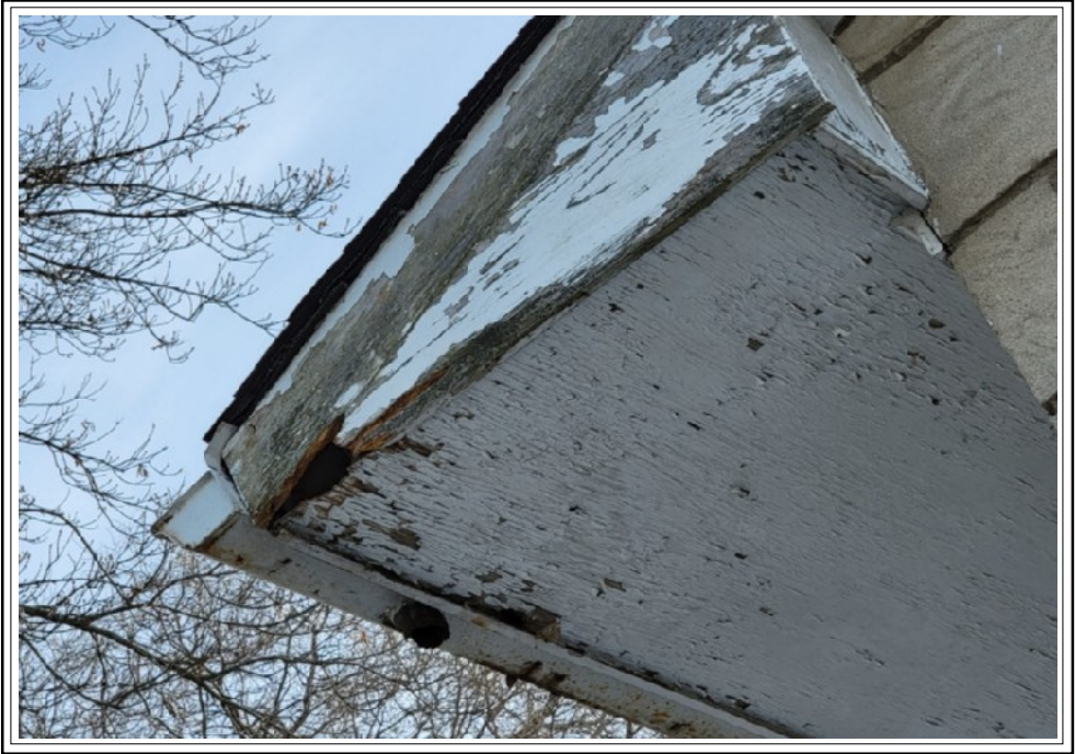
Defective Soffits & Fascia Evidence of Possible Rodent Infestation
