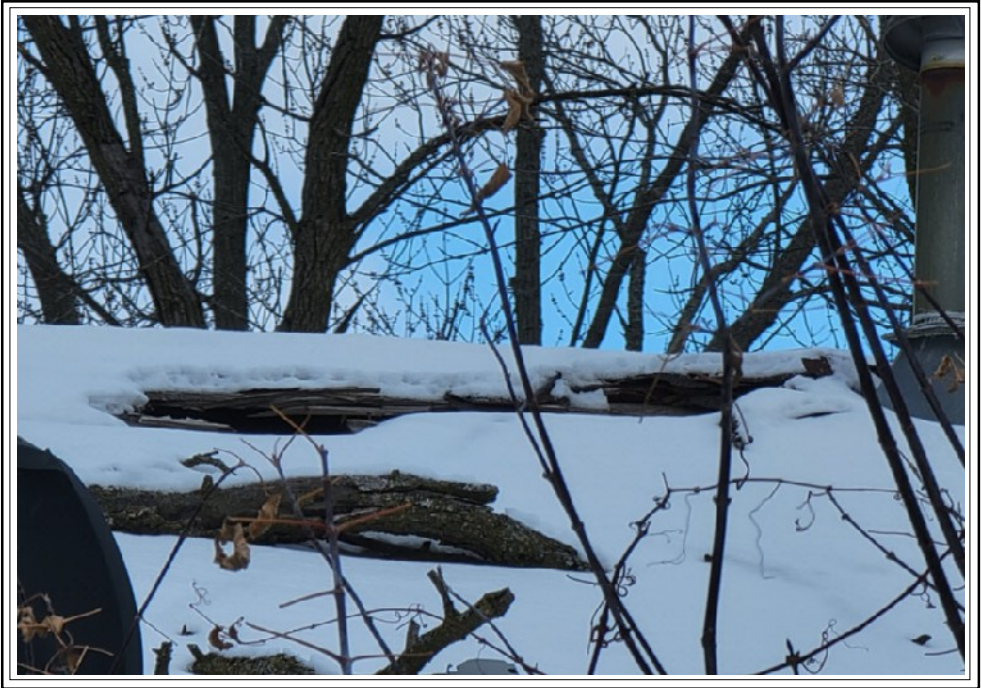
Defective Roof Evidence of Infiltration of Elements/Vermin
