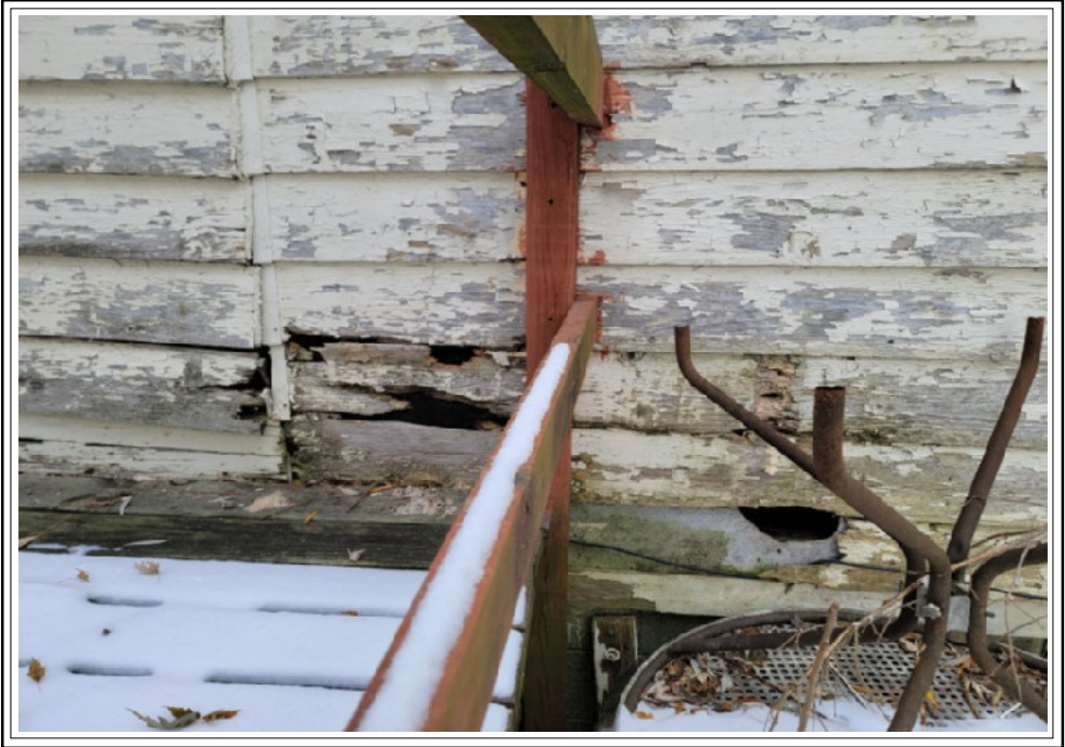
Defective Siding Evidence of Infiltration of Elements/Vermin
