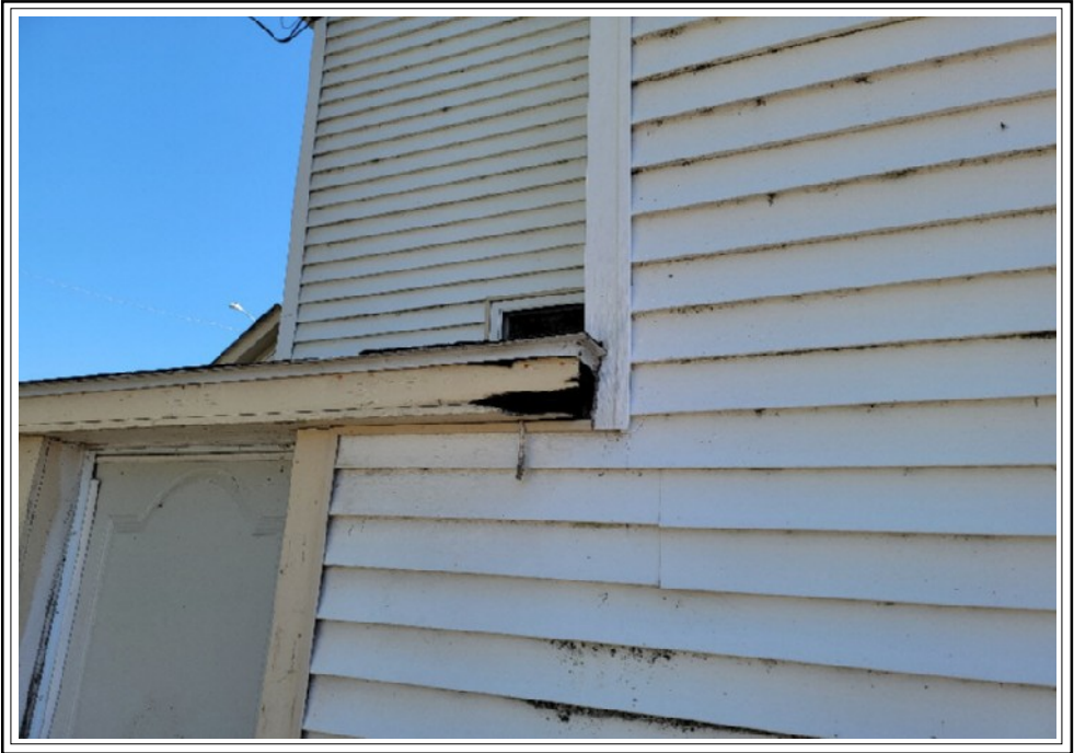
Defective Soffits/Fascia
