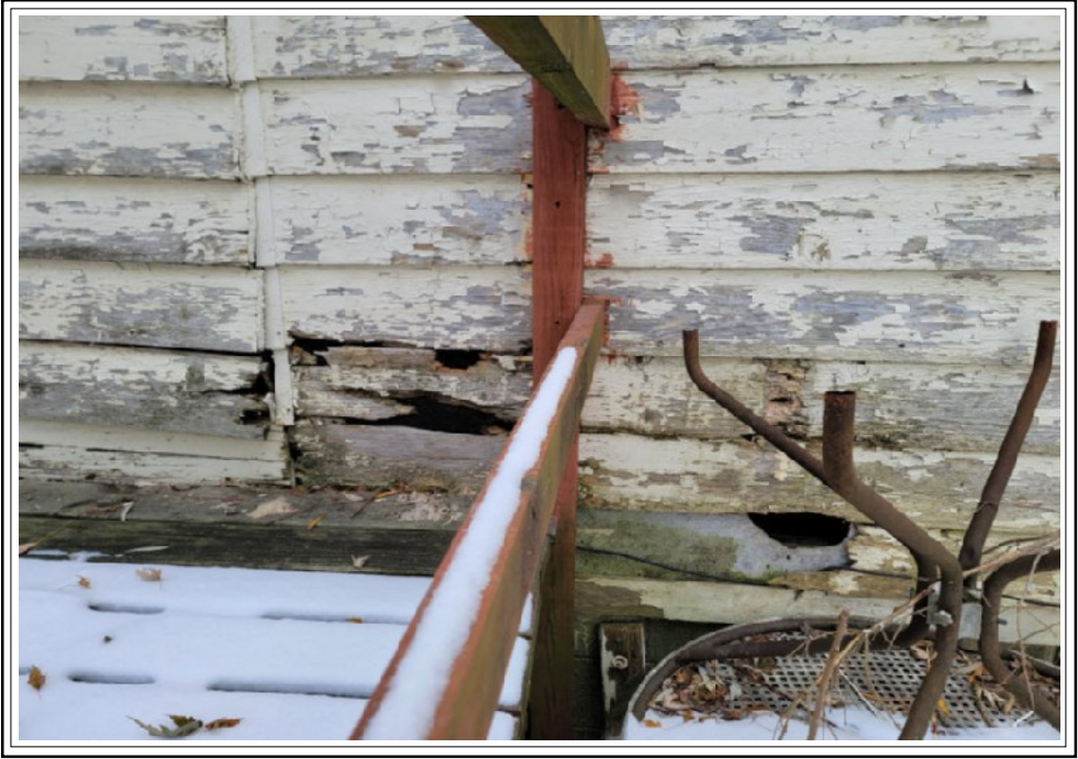
Defective Siding Evidence of Infiltration of Elements/Vermin
