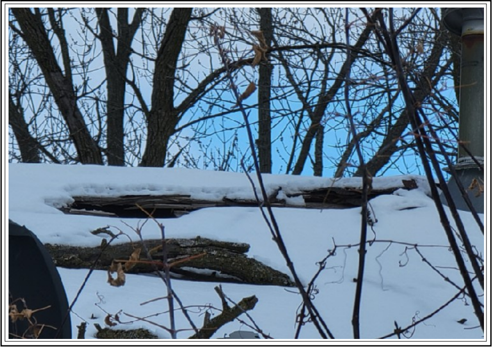
Defective Roof Evidence of Infiltration of Elements/Vermin
