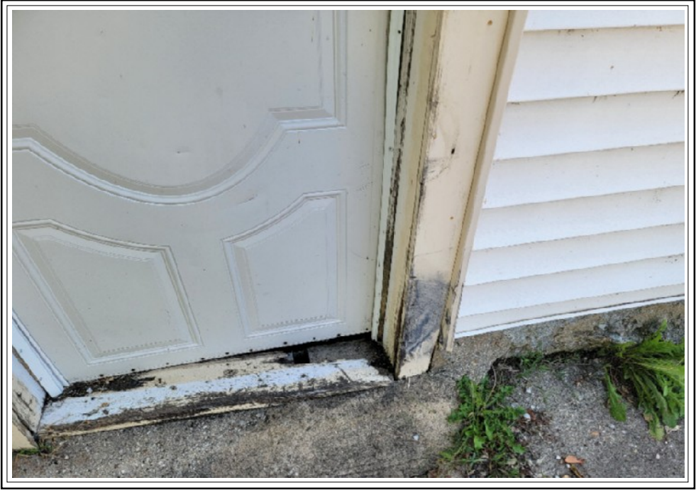
Defective Door Sills/Jambs
