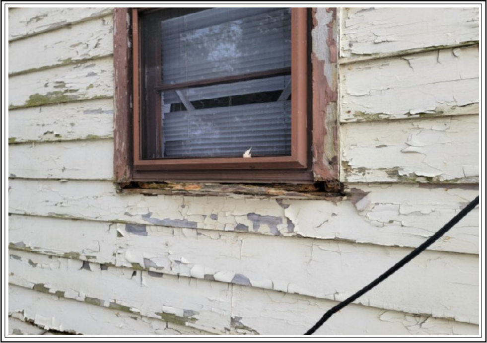
Defective Window Sills/Casing Evidence of Infiltration of Elements
