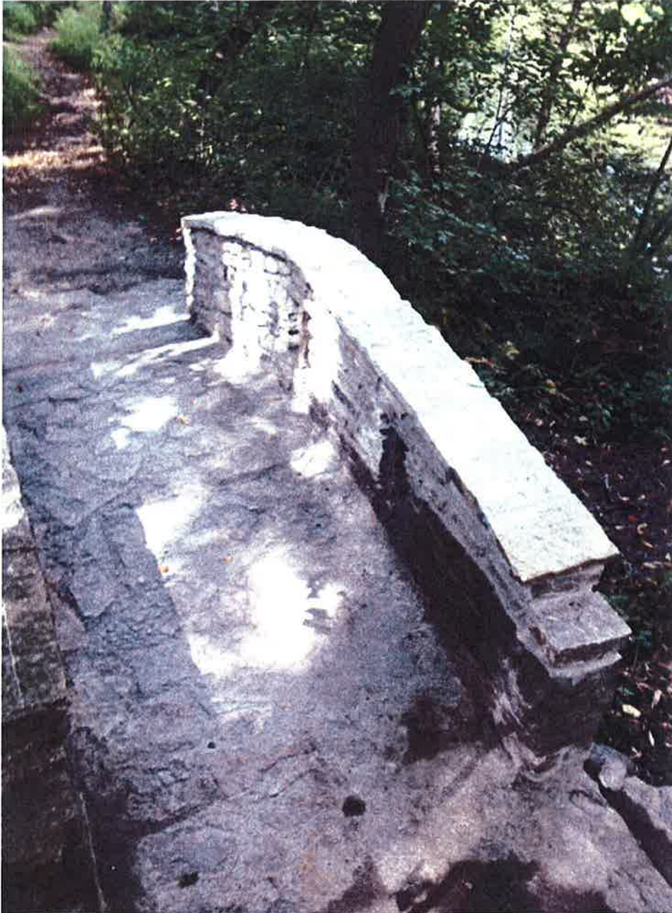
Restored bridge, right side railing had to be 80% rebuilt from scratch.
