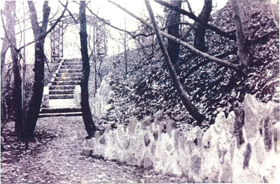
WPA trail project (1937) bridge that was restored center left in photo.
