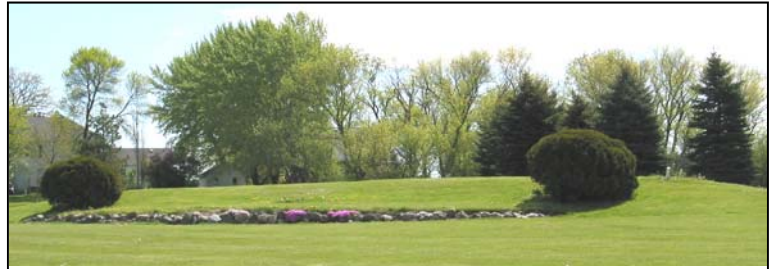
A mound dispersal cell with spruce trees serving as a backdrop on the upslope side of the mound. The field stone accent wall on the downslope toe of the system provides an area to plant perennial flowers like creeping phlox. The globe yews are actually planted in the downslope toe of the mound, but are well away from the distribution piping network.
