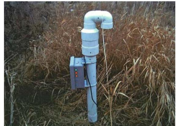
*Septic Tank Heating Device*
