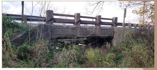
► The bridge sufficiency rating is a numerical value computed from many factors to include the condition of the bridge. A bridge with a sufficiency rating of 100 is in perfect condition. Bridges with a rating less than 50 are eligible for replacement funding.
