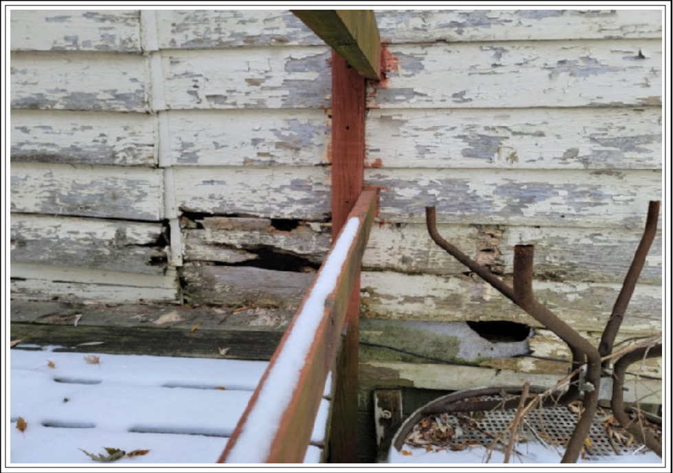
Defective Siding Evidence of Infiltration of Elements/Vermin
