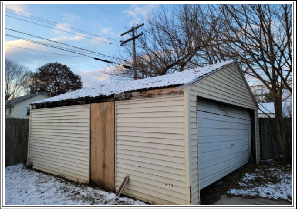
Defective Garage Components Roof, soffits/fascia, door
