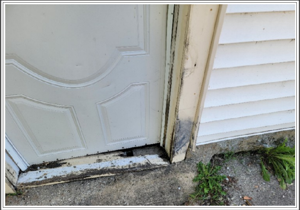
Defective Door Sills/Jambs
