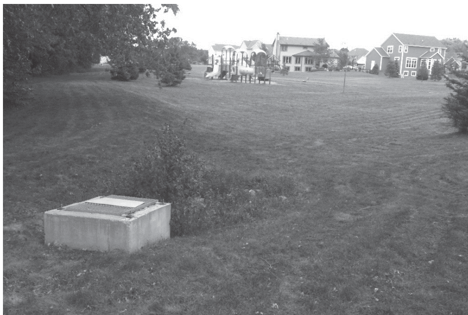
A dry detention basin serving a residential subdivision in Greendale, WI.
